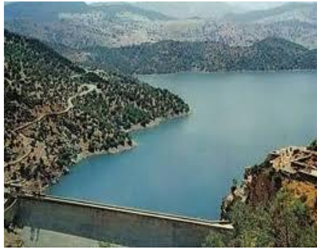
Figure 3. Oued Fodda concrete gravity dam
