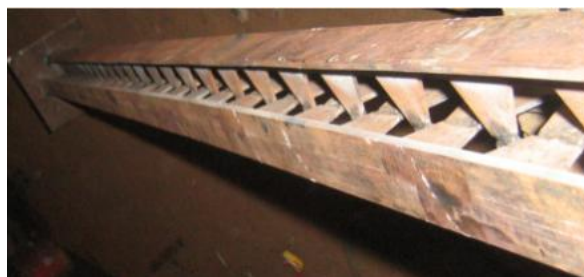
Figure 3. Built-up castellated cruciform steel column
