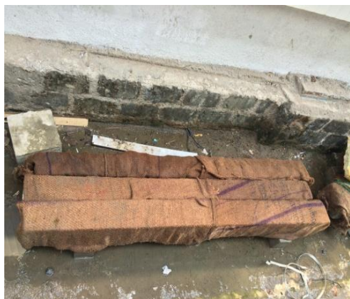
Figure 5. Curing of beams
