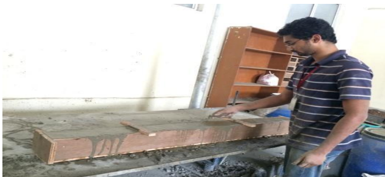
Figure 4. Casting of beams
