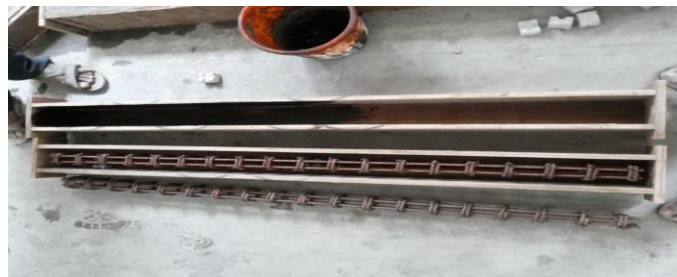
Figure 3. Moulds and reinforcements for beams
