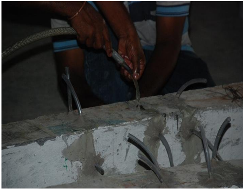
Plate 5. Injecting the epoxy resins into pipes
