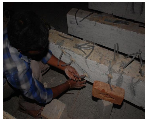
Plate 2. Fixing the PVC pipes into the grooves
