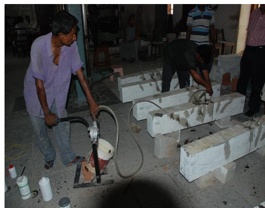
Plate 4. Injecting the epoxy resins into pipes
