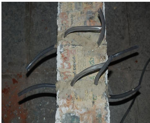
Plate 3. Fixed the PVC pipes into the grooves
