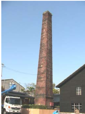
Figure 5. Appearance of the chimney
