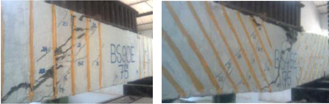
Figure 2. Crack pattern of specimen in series S2
