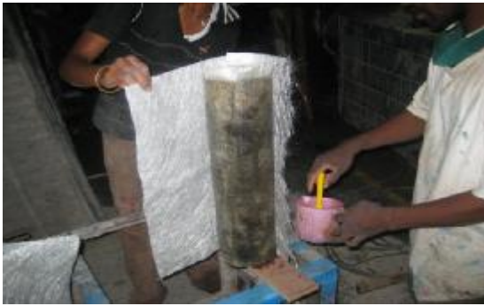
Figure 4. Wrapping under progress
