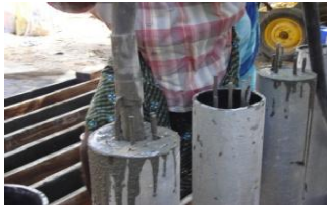
Figure 3. Casting under progress
