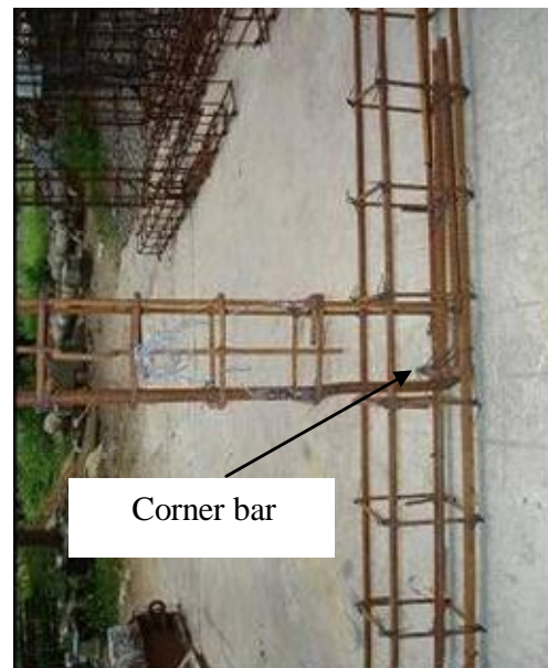
Figure 2. View of reinforcement grills with corner bars
