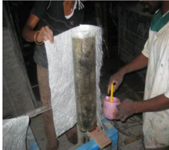
Figure 2. Wrapping under progress
