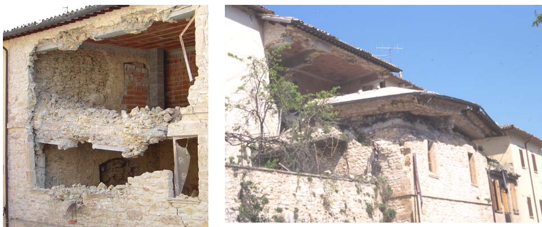
Figure 1. Example of a) Out-of-plane collapse of a wall with r.c. tie beams, b) roof hammering the masonry walls
