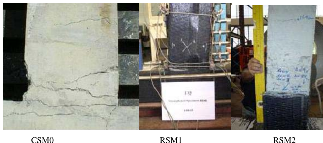
Figure 9. Ultimate failure of specimens CSM0, RSM1 and RSM2.
