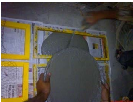
Figure 3(a). Placing of mortar into moulds
