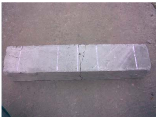
Figure 9. Failure pattern of fiber reinforced concrete prism
