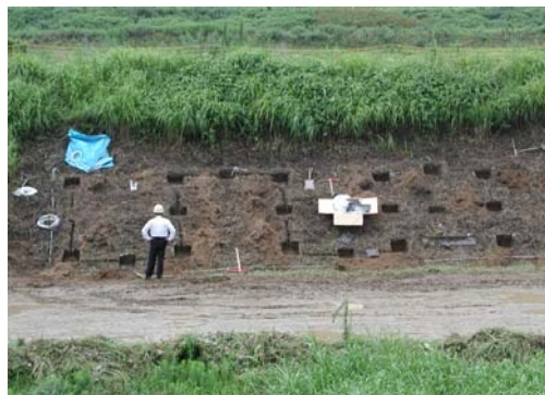
Figure 3. Installation of optical fibers
