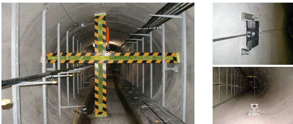
Figure 8. Installed condition of optical fiber sensors
