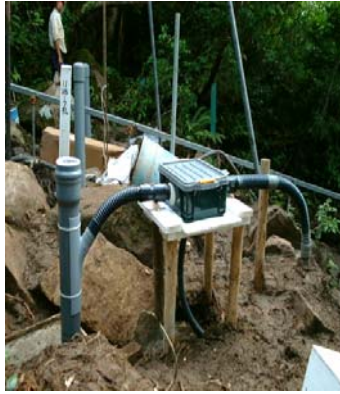
Figure 10. Installation of optical pipe strain meter
