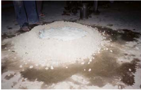
Plate 1. Mixing of polymer cement concrete
