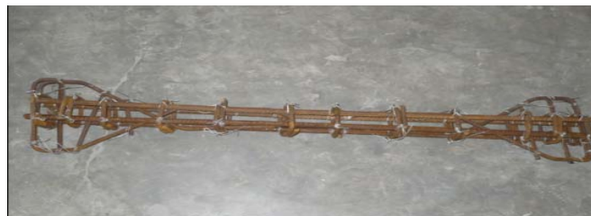
Figure 2. Reinforcement cage for short column
