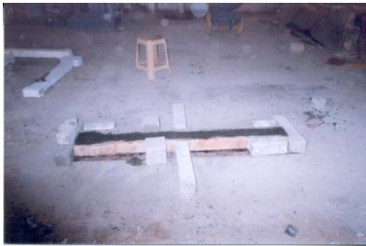
Figure 3. Casting of test specimen
